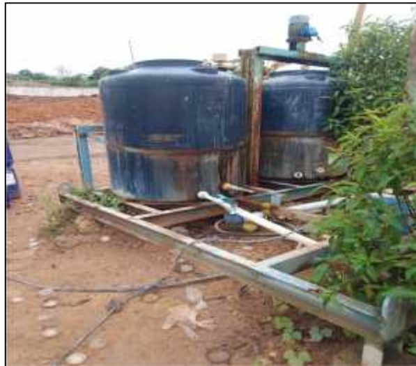
Gambar 4.4. Bak Penampung Chemical Organic Coagulant
