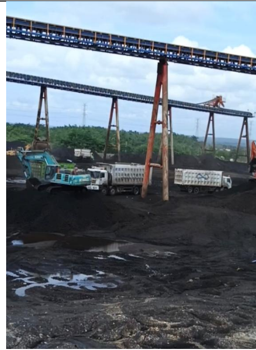
Gambar L.1 kondisi area stockpile
