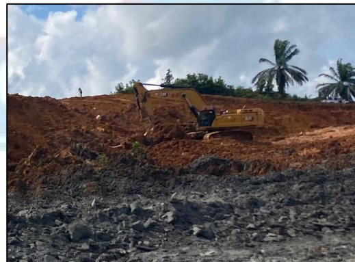
Gambar D.3 Loading Top Soil
