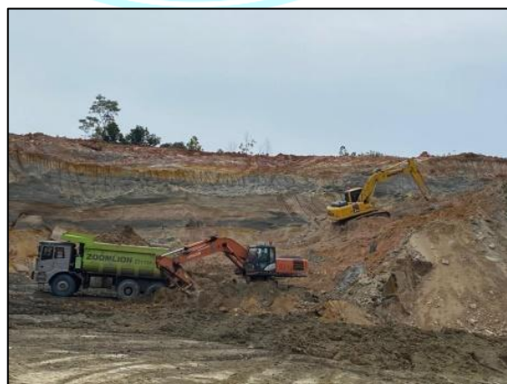
Gambar 4.6 Loading Material di Area Lereng
