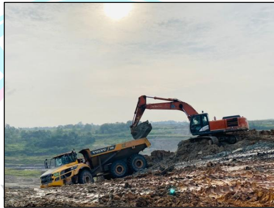
Gambar 4.7 Pengupasan Material di Area Lereng Miring
