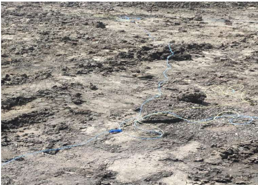
Gambar C.6 Tie Up (Perangkaian Lubang Ledak Surface Delay )
