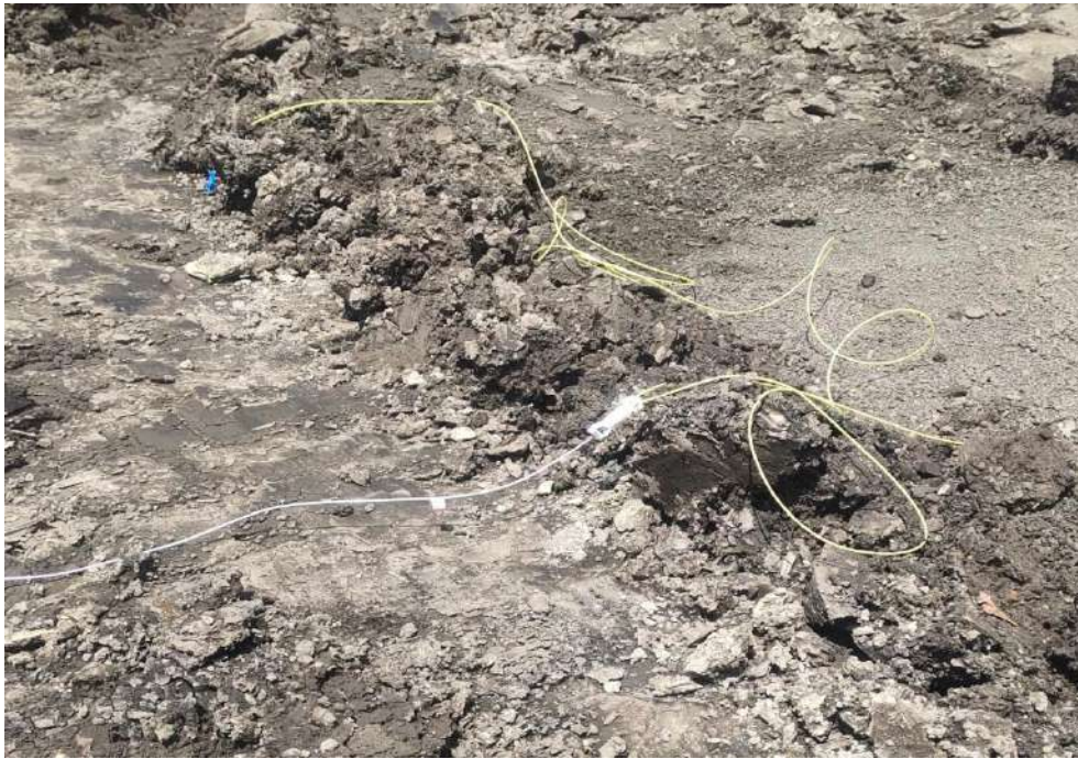
Gambar C.5 Tie Up (Perangkaian Lubang Ledak In-Hole Delay )
